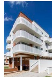
Residential construction and renovation - Trnava, Slovakia
