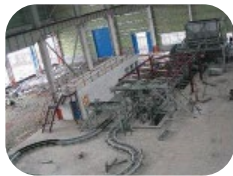
Construction of the foundry commenced
