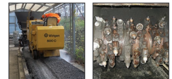
Milling the reinforced area
